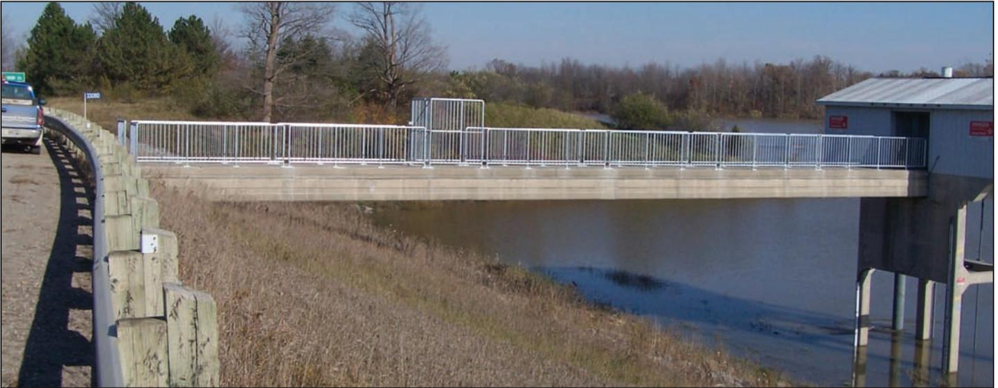
Railings were installed in 2008 on the catwalk to the Parkhill Dam control building. A locked gate was also installed to prevent unauthorized access.
