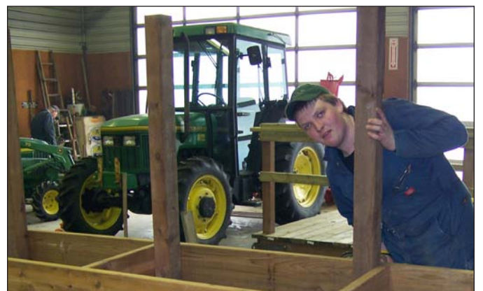
Co-op student Greg Urquhart acquires carpentry skills in 2011 while helping build Morrison Dam Conservation Area fishing dock.
