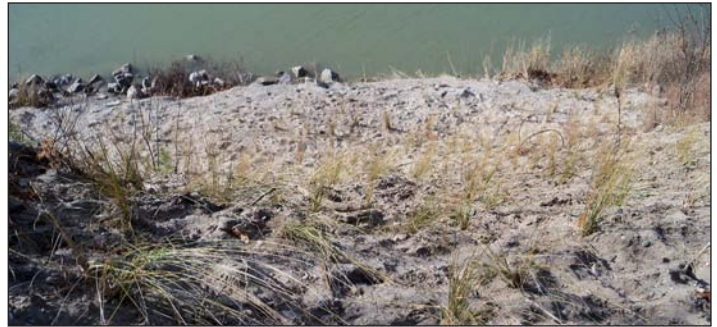
Port Franks erosion control repairs (below water's surface) reinforced the integrity of the shore wall.
