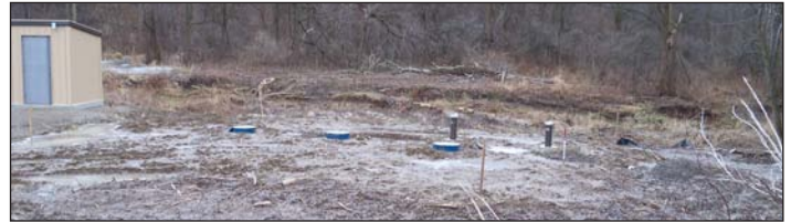
Site preparation for an integrated climate change monitoring station in Parkhill began in 2011. (Photo above was taken in January 2012).
