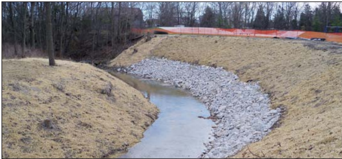
Repair following bank failure at Walker Drain was among 2011 Water and Erosion Control projects.
