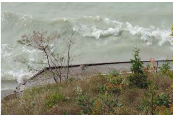
Steel Walls at base of steep slope
