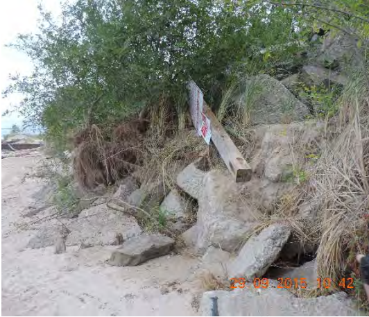
Dumped concrete rubble and stone.
