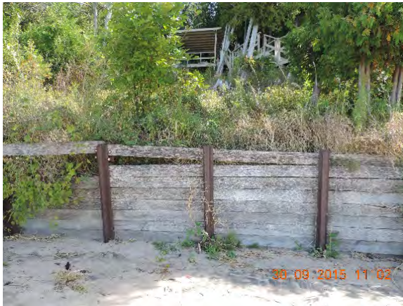
Deteriorated wooden frames.
