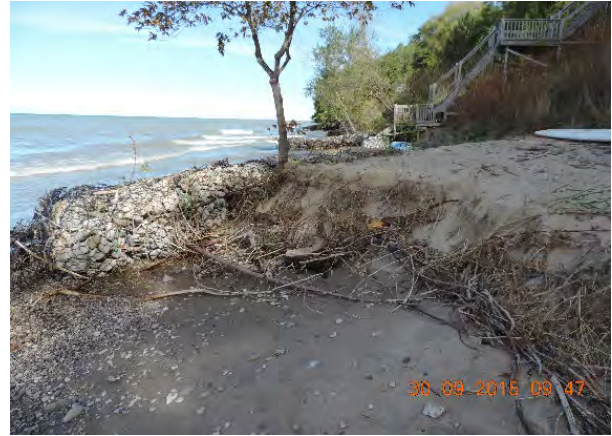
Outflanked and deteriorated gabion baskets.
