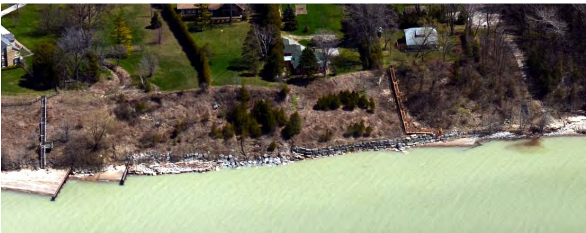
Ad-hoc, inconsistent, piecemeal shoreline protection works.
