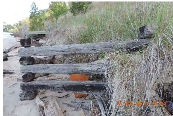
Deteriorated structures, emptied of materials.
