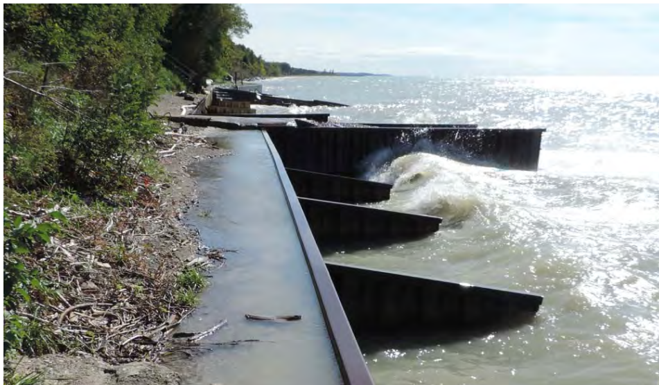
Wave Overtopping and ponding behind structures.
