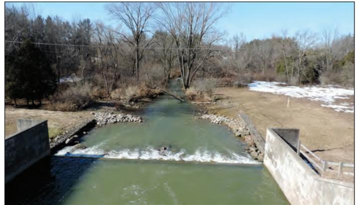
The photo at left shows a project, at Stewart Gully, to stop gully erosion that might otherwise impact a municipal road. Above, the photo shows Morrison Dam after flooding moved some protective riprap that was out of place.
