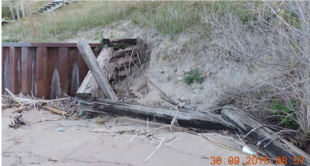
Flanking and lack of coordination between properties of shoreline protection works.
