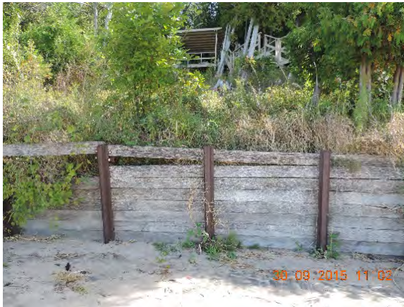
Deteriorated wooden frames.
