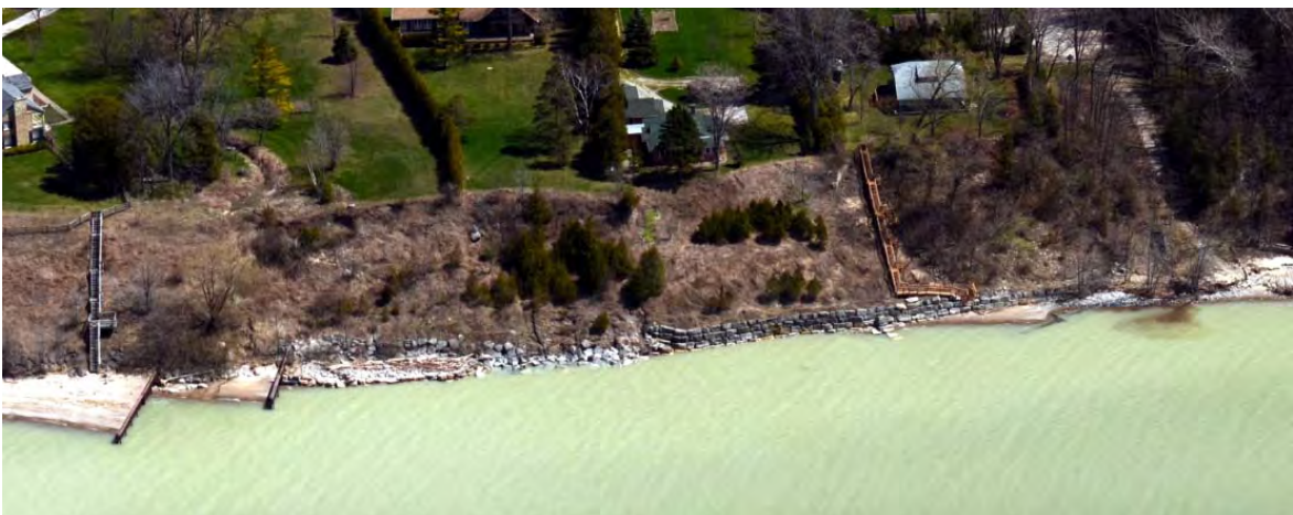
Ad-hoc, inconsistent, piecemeal shoreline protection works.
