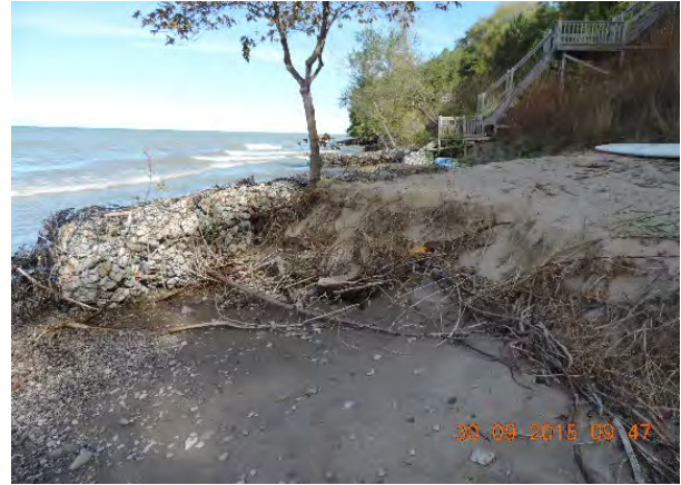
Outflanked and deteriorated gabion baskets.
