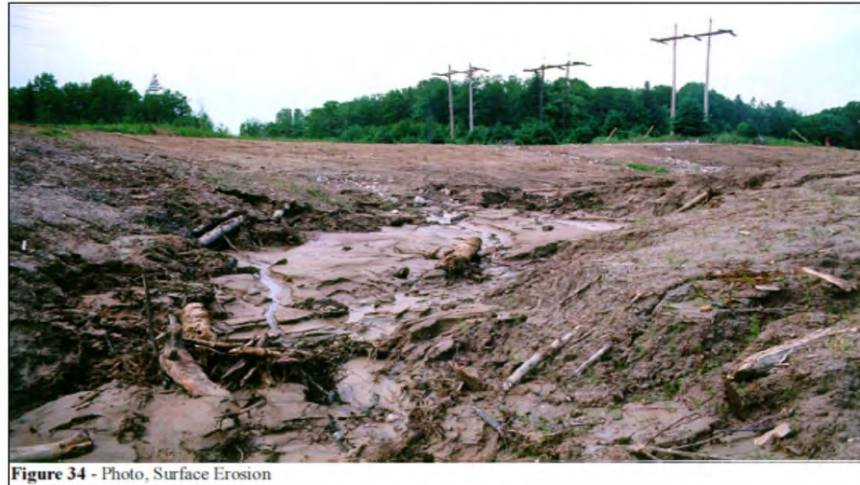
Figure 7.4: Surface Drainage Issues, From MNRF – Figure 34, Terraprobe, Geotechnical Principles for Stable Slopes (1997) Page 37
