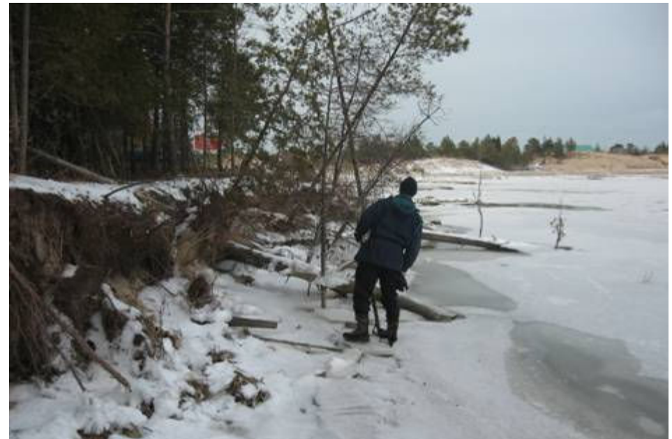
Photo P45 (13-Dec-07): Bank erosion downstream/south of southern end of revetment.
