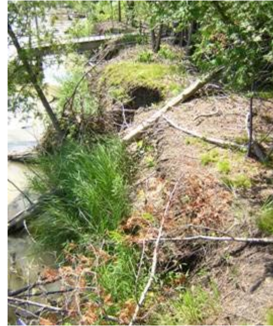
Photo P43 (25-Jul-08): Bank erosion downstream/south of southern end of revetment.
