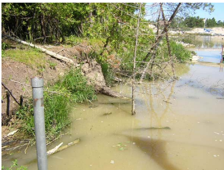
Figure 3 – Potential Bank Erosion (approx. 35 m downstream (south) of Weir G, photo looking north)
