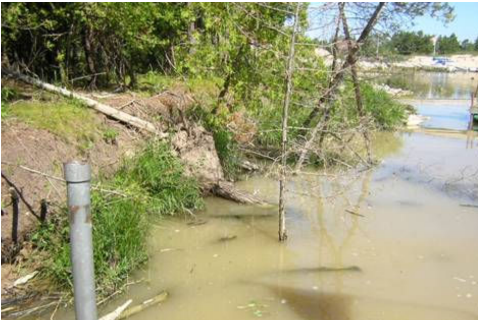
Photo P44 (25-Jul-08): Bank erosion downstream/south of southern end of revetment.
