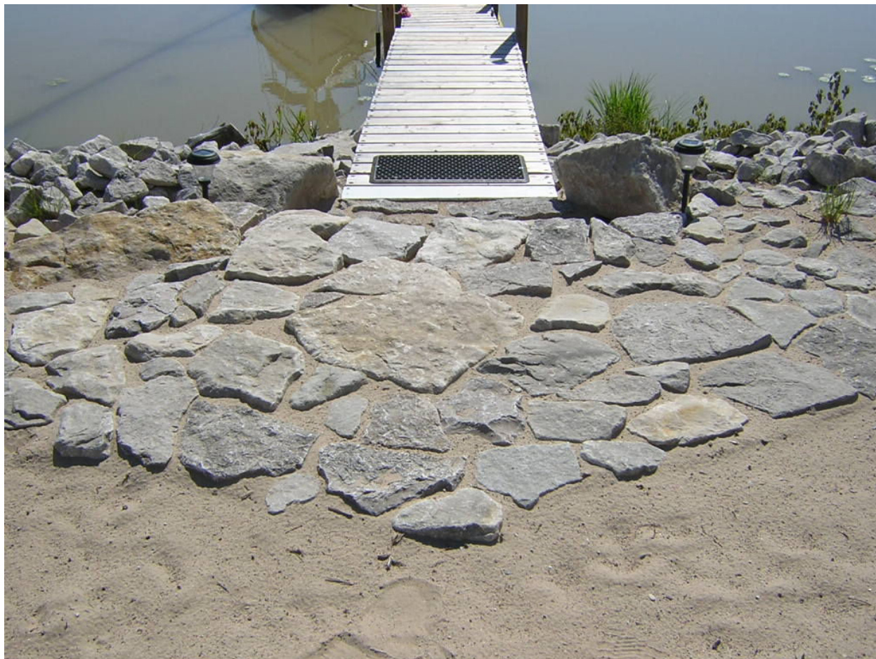
Figure 4 – Evidence of Rock Displacement by Local Residents (between Weir D and Weir E)
