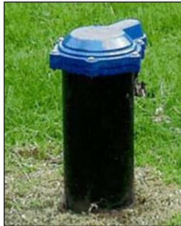
A properly-maintained wellhead can limit potential pathway for pollutants to reach groundwater sources.
