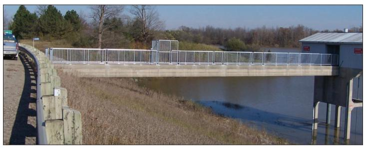
Railings were installed in 2008 on the catwalk to the Parkhill Dam control building. A locked gate was also installed to prevent unauthorized access.
