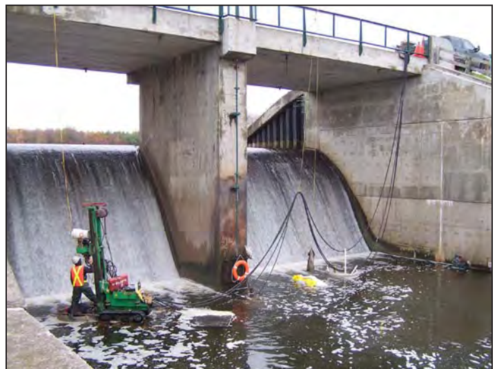
Upgrade work at Morrison Dam in 2006.
