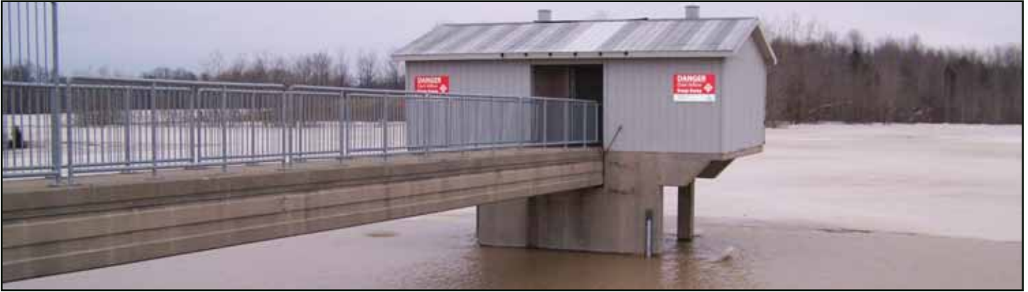
Parkhill Dam control building is shown at reservoir during time of high water.
