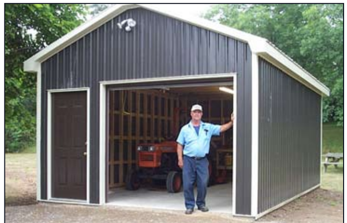
Rock Glen Conservation Area Supervisor Dale Cable at the new maintenance building.
