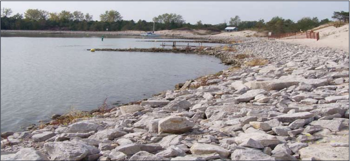
The Armstrong West erosion control project was a significant undertaking and was completed in 2007.
