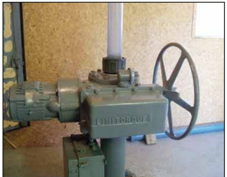
Photo above shows the refurbished controller at Parkhill Dam.
