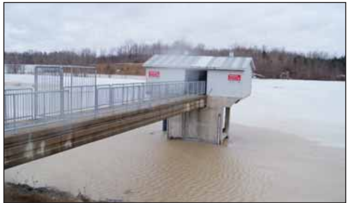
The photo above shows the Parkhill Dam control building and Parkhill Reservoir on March 13, 2010, during a period of high water.
