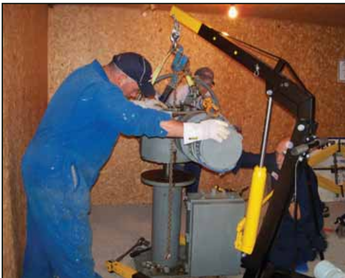
Photo above shows the removal of Parkhill Dam controller for refurbishing.
