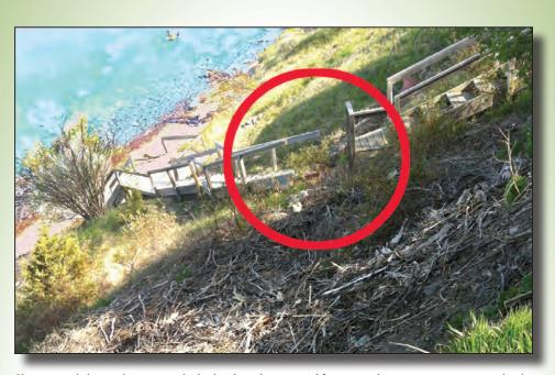
Slope instability indicators include displaced posts and fences, poles, monuments, guardrails, broken or displaced retaining walls, and stairs, among other indicators mentioned in this fact sheet. Please read the Recommended Management Practices panel inside.
