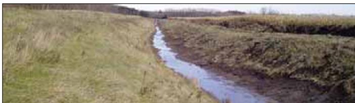
The above photo shows the 2013 cleanout of sediment in the bottom of the Cameron-Gillies Diversion Channel located in the Municipality of North Middlesex.
