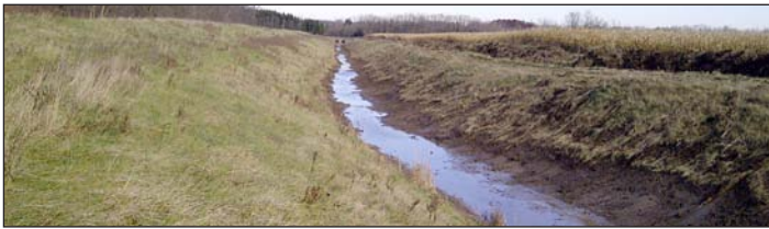
The above photo shows the 2013 cleanout of sediment in the bottom of the Cameron-Gillies Diversion Channel located in the Municipality of North Middlesex.
