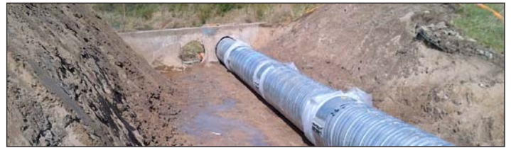
Above photo shows 2013 repair work on the control structure for the Cameron-Gillies Diversion Channel.
